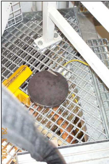
Azimuth bogie hard point in level 3 floor
