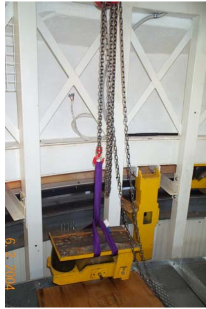
Replacing Bogie: Block and tackle-Sling arrangement
